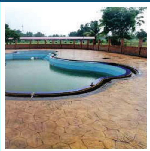
CONCRETE IMPRINT ON POOL DECK
